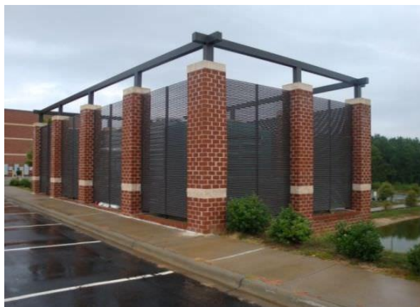
Screening of Urban Utilities at India Habitat Centre
